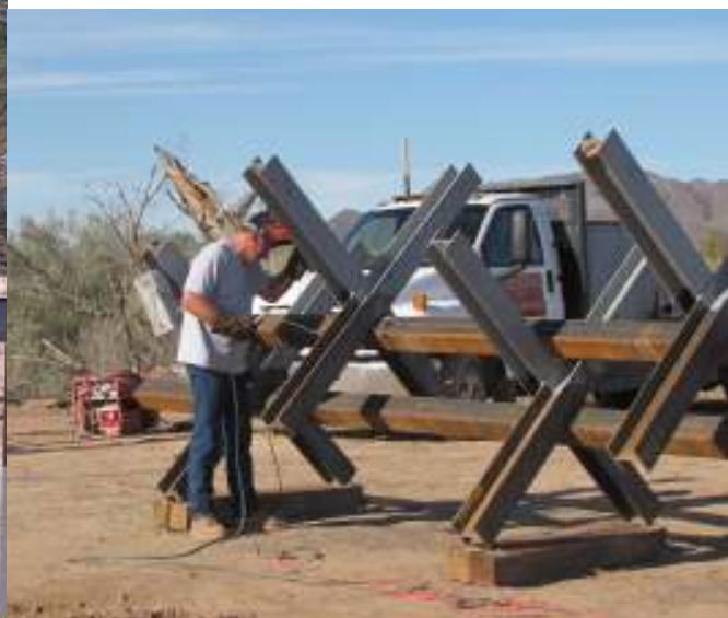
Fit is the most important part of the equation as is demonstrated by Mr. John Jarvie (left) adjusting this mid-rail connection before he “tacks” it together. (Below) Jim Ranard ready to put a bead on a section of Normandy style fence
