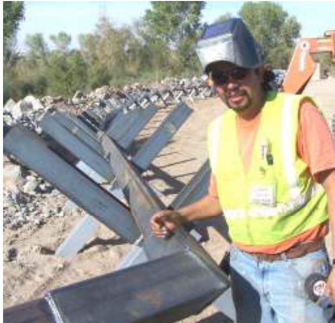
(Left) Jose Hurtado as he completes the installation of a field fabricated transition fitting on Type II Normandy style fencing. (Below) close up view of welded connection.
