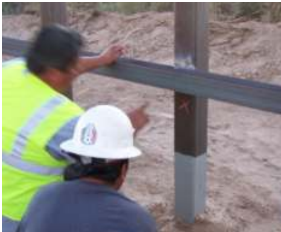
(Above right) Typical mid-rail welding connection. (above left) Jose Hurtado watches as Oscar Galindo inspects a mid-rail welded connection. Each weld is inspected for proper size, penetration and final removal of slag.
