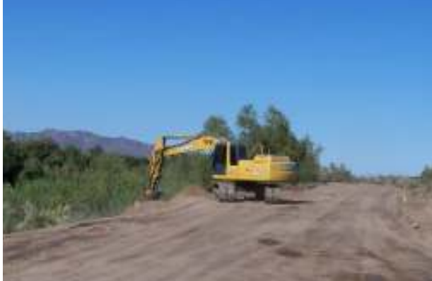
Preparing the embankment for Rip-Rap
