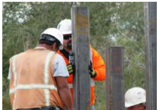
(Right) Jeff uses a level just to double check the old eyeball, yes Jeff, its plumb!
