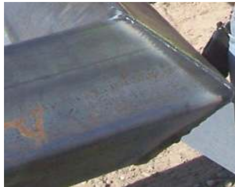
(Left) Jose Hurtado as he completes the installation of a field fabricated transition fitting on Type II Normandy style fencing. (Below) close up view of welded connection.
