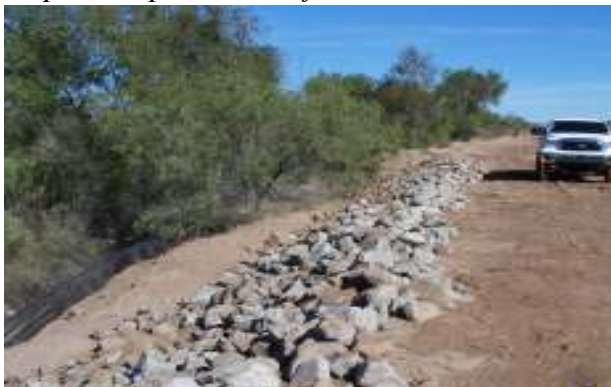
Completed section ready for inspection
