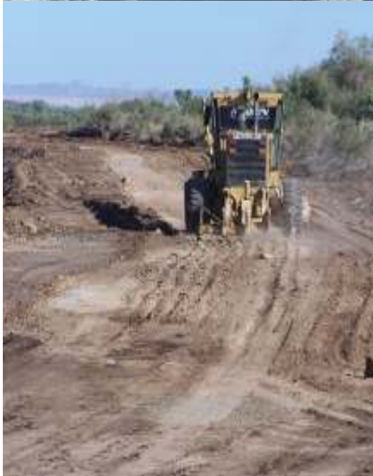
(Above) a Caterpillar Model 140 H blade grader rips the future roadway as it begins to process the soils for optimum compaction
