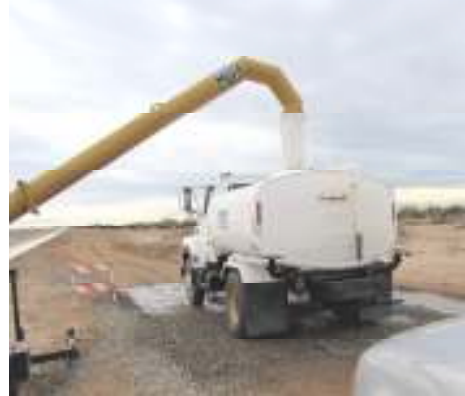
The pump (left) is a diesel operated 14” centrifugal single stage unit and was set into the Salinity Canal near the construction area on October 22, 2008. Water was delivered to the construction area using water trucks. (below) a water truck “filling up” at the pump
