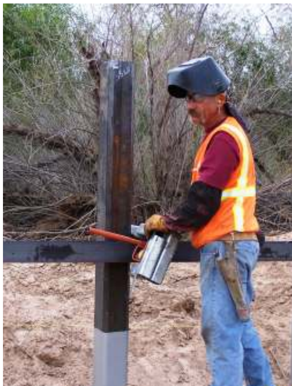
Fit is the most important part of the equation as is demonstrated by Mr. John Jarvie (left) adjusting this mid-rail connection before he “tacks” it together. (Below) Jim Ranard ready to put a bead on a section of Normandy style fence
