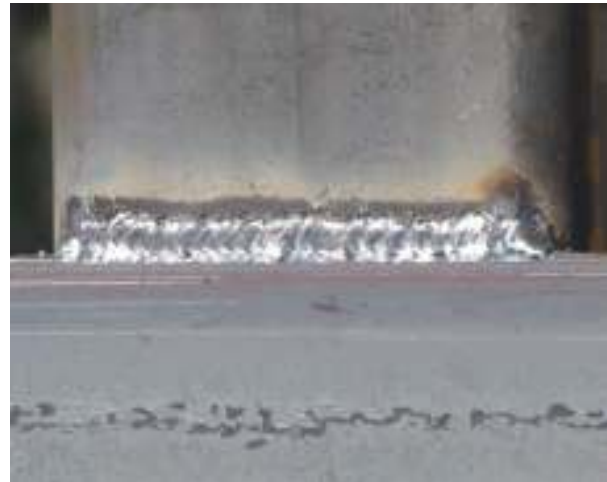
(Above right) Typical mid-rail welding connection. (above left) Jose Hurtado watches as Oscar Galindo inspects a mid-rail welded connection. Each weld is inspected for proper size, penetration and final removal of slag.
