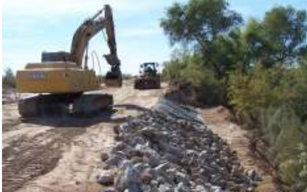
In process placement of materials
