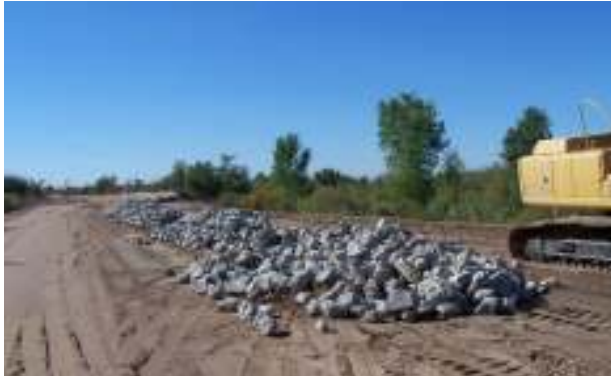
Stockpiled materials await placement
