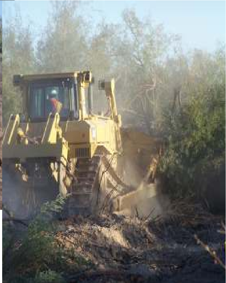
(Above) a Caterpillar Model 140 H blade grader rips the future roadway as it begins to process the soils for optimum compaction
